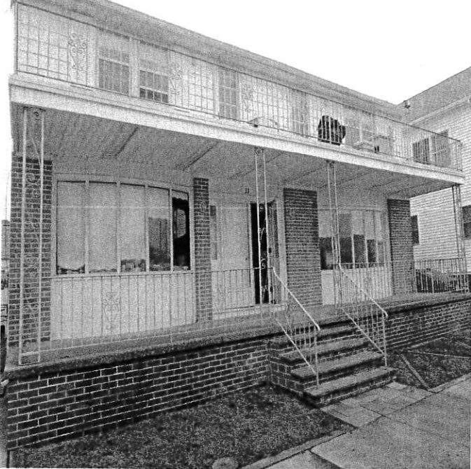
Front View Date Taken:12/18/2012
